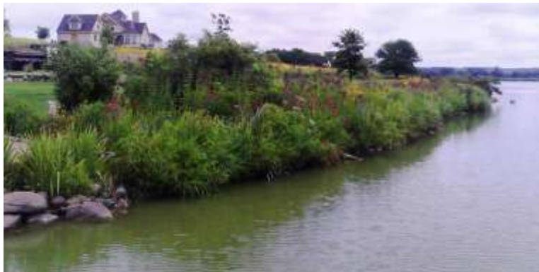
Figure 47: Completed native planting (photo from HealthyLakesWI.com)
